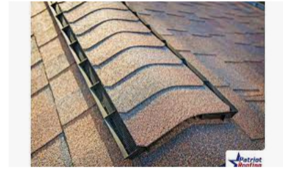
The Ridge Vent: A Look at Its Advantages patriotroofing.com
